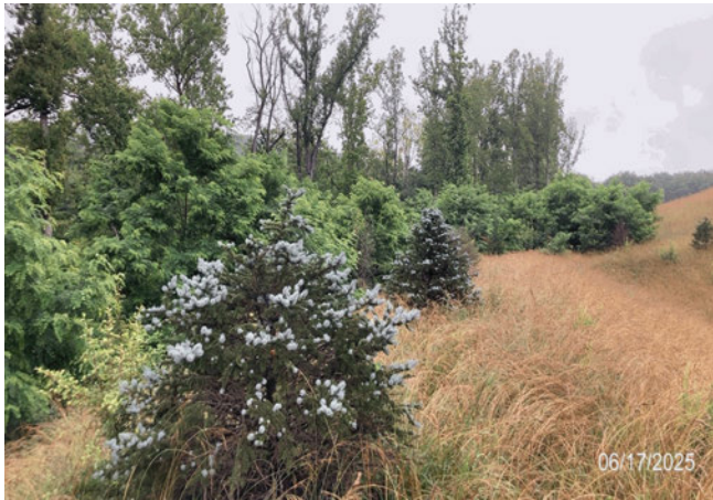
Remove all woody vegetation from the embankment.
