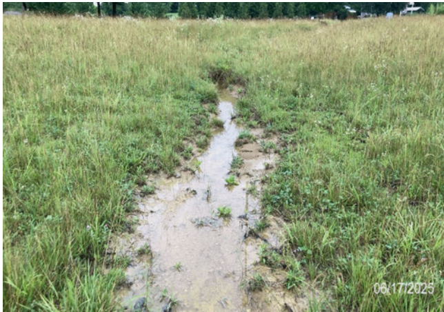
Repair and stabilize eroded areas within the southeast inflow channel. Apply seed and straw mulch to all bare areas once repairs are complete.
