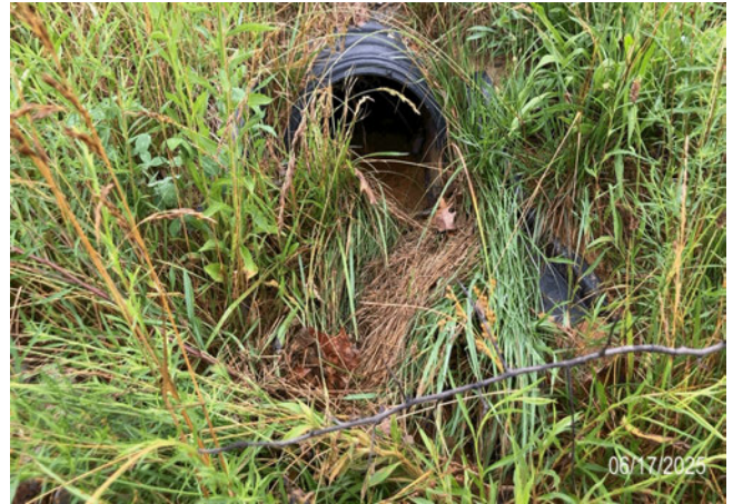
Remove accumulated sediment from within and below the northwest inflow pipe.
