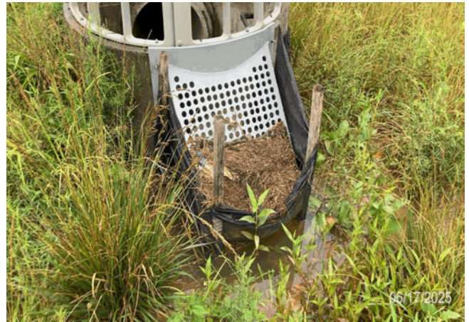
Remove silt fence from around the debris rack.
