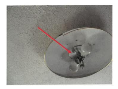
The Light Shield on the living room light fixture was found to be Asbestos Containing by the laboratory.
